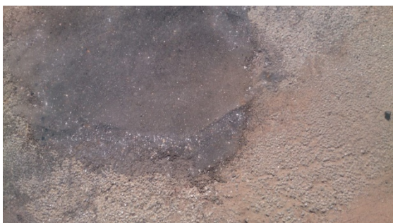
Fill pothole and compact level to existing road
