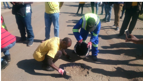
Clean hole from dust and apply liner coating
