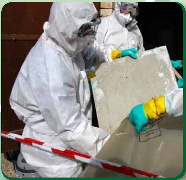
Professional workers in their protective personal equipment handling asbestos waste
