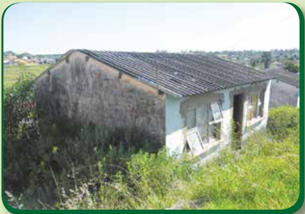
An image of asbestos wall sheeting corrugated
