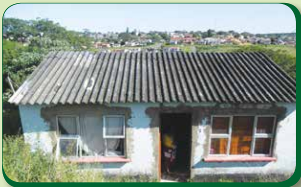
An image of cement-asbestos corrugated
